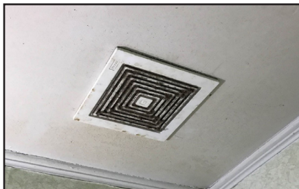
Left: A moldy exhaust fan observed in a Sullivan County hotel/motel in October 2016. Right: The same fan observed in April 2019.
