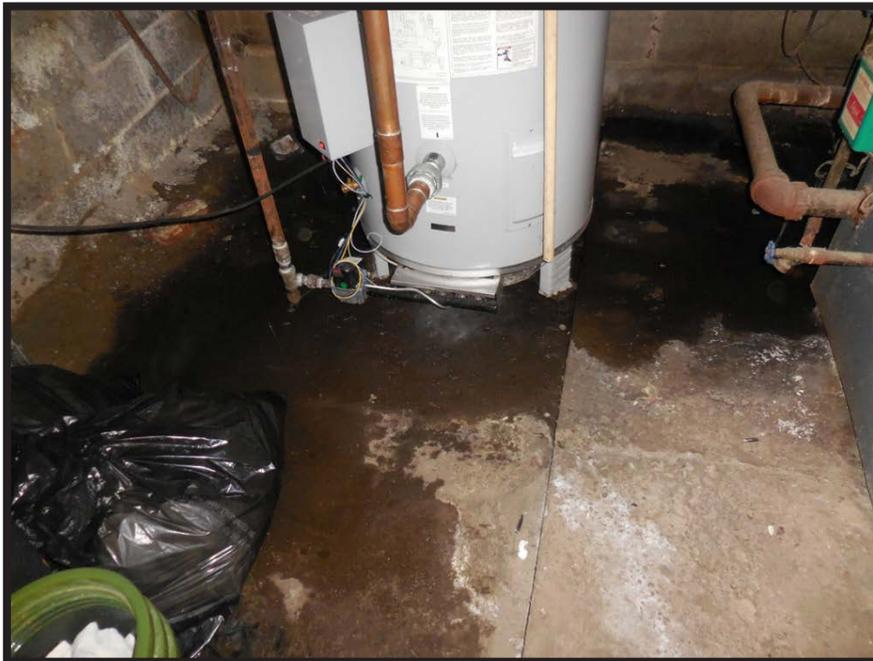
Leaking pressure release valve
