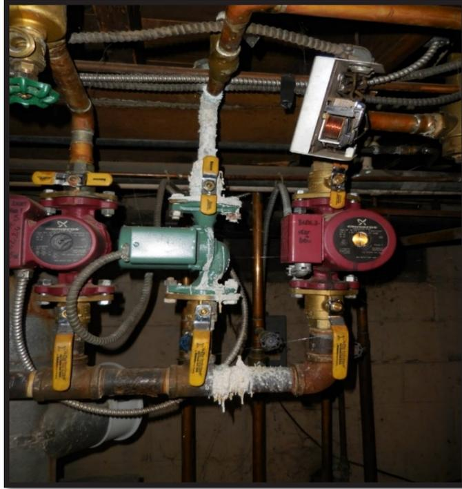
Corrosive build-up on boiler pipes
