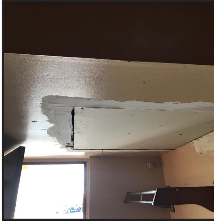
Water damage to ceiling in room with improper repair
