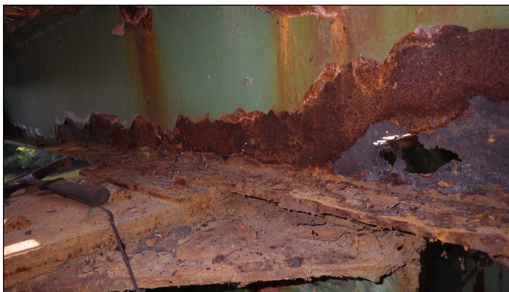
Floor Joists on Approach Spans
